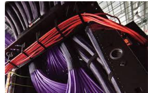
Cable Management and Cabinet
